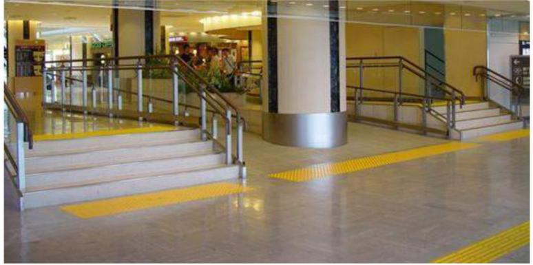
**Figure 11.2: Warning Blocks** **Figure 11.3: Placement of warning blocks for steps**
